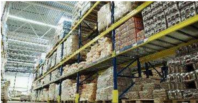
Chemical, Food & Pharma Warehousing
